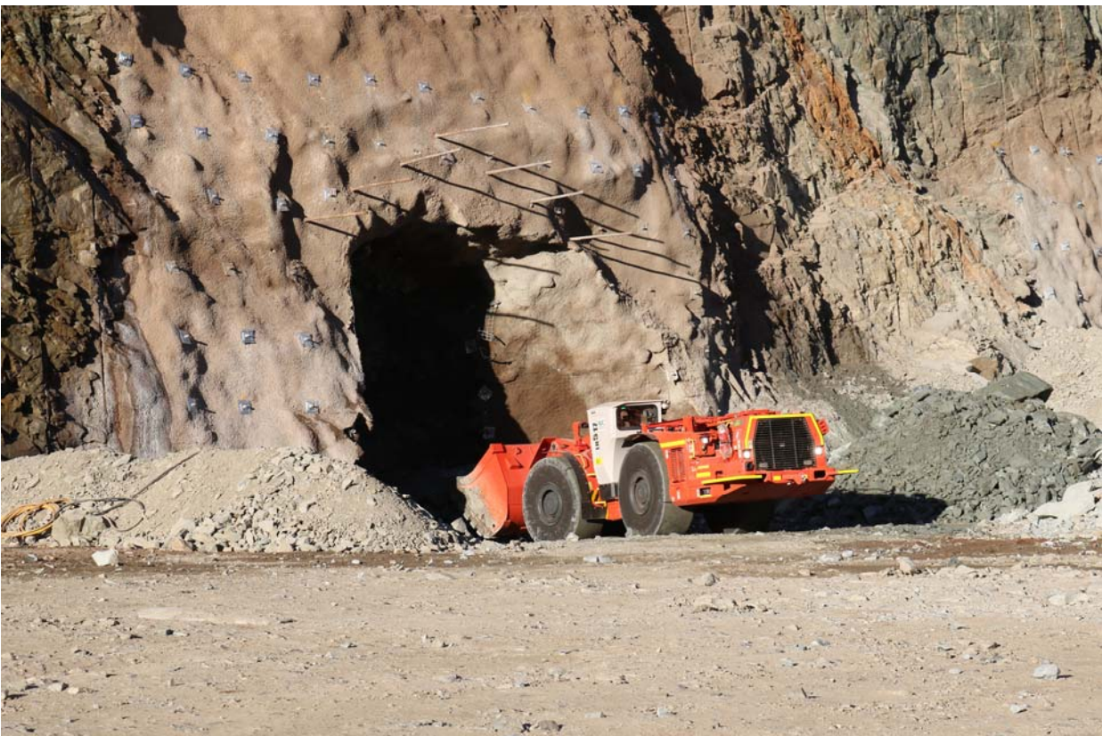
Figure 1: First mining of Beresford's portal from the base of the Westralia open pit.
